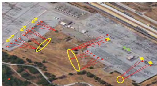
Equipment with gunshot damage
